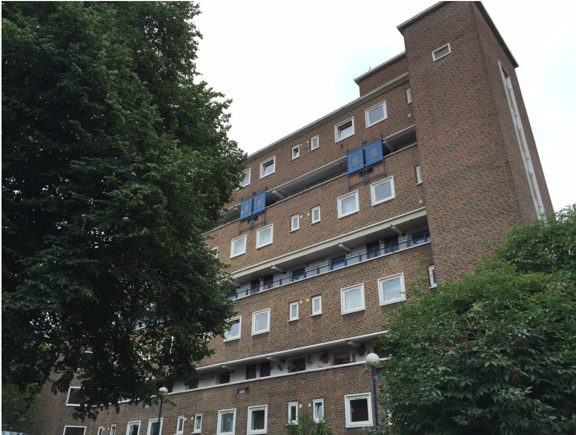
Image 3: Northeast (rear) elevation of the building from Elizabeth Street
