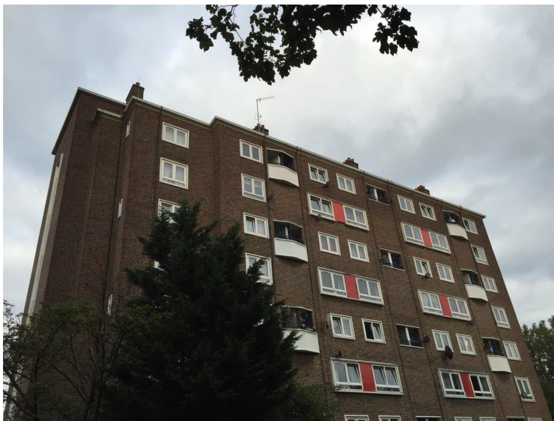
Image 2: Closer view of the building from Elizabeth Street (Southwest elevation)
