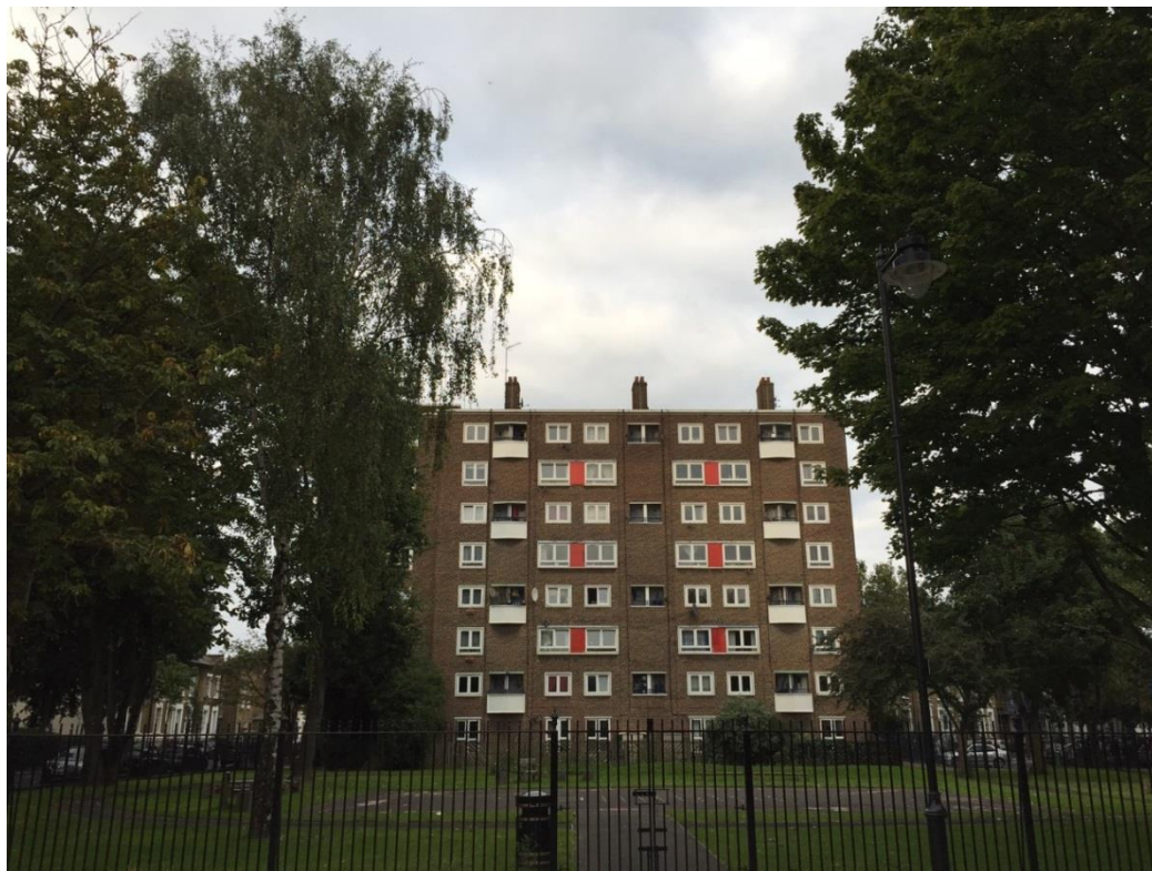
Image 1: View of the building from Rotherfield Street (Southwest elevation)
